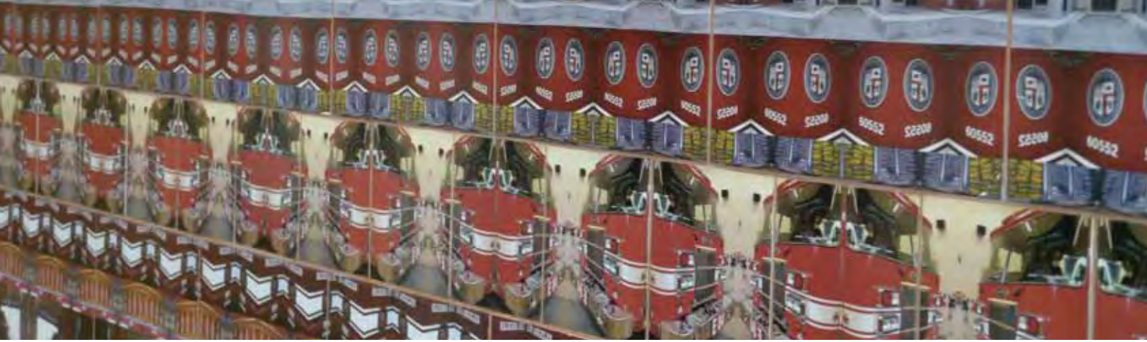
(Top) Los Angeles County Fire Department/ Woodland Hills Station, Woodland Hills, CA "Ladders," 2009
